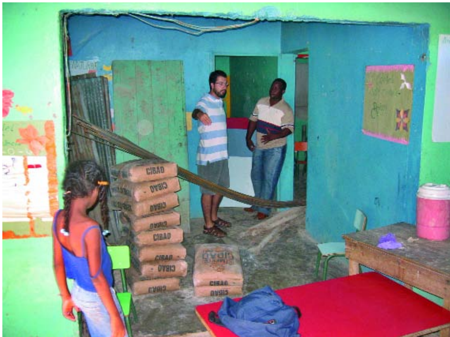
Oriol Regales overseeing the construction of a house.
